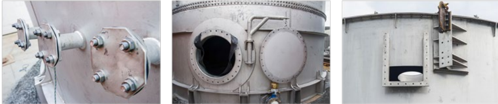
Figure 11 – Albion Leach Reactor Nozzle and Penetrations
